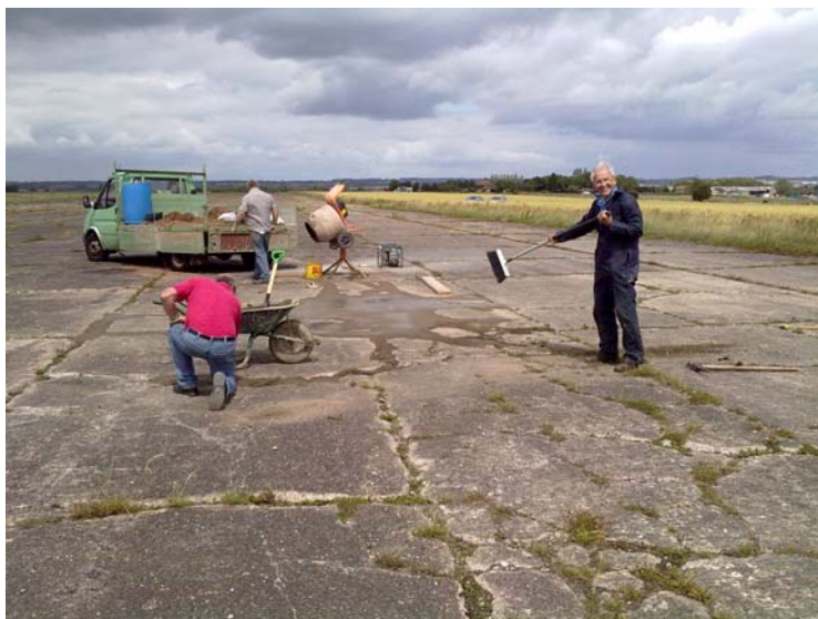
Melton Airfield restoration work being undertaken by club members
